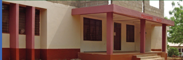
PARTIALLY COMPLETED MEN'S DORMITORY
